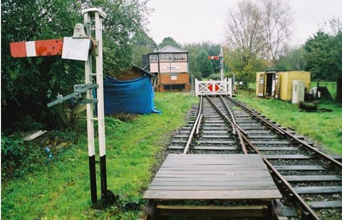
General view of site: Pavilion on left, visitor van on right, signal box in distance
