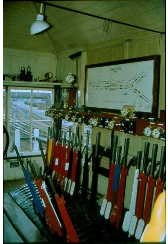
Two views of the interior of Redbridge Signal box, 21 October 1978
